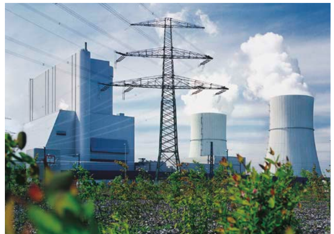
Fig. 11 SIPROTEC 4 in power plant application
